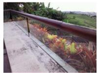
CONDITION: Overall, satisfactory condition, Secure, Weather wear at the main lanai railing. Refinish maintenance
