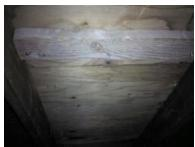
COMMENTS: The roof structure appears very solid. No Hurricane ties at rafter/wall connections, steel
