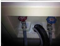
VALVES: Supply valves appear O.K. No leaks or major corrosion.
