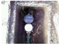
WATER METER FLOW DIAL: The Flow Dial at the water meter with normal dial movement, normal for pool and pond
