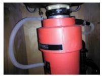
CONDITION: Operational and appears satisfactory, No rust at blade or sink connection. Disposal safety rubber boot is needed at the sink drain.
