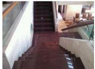
Hallway stairs are in overall, good condition. Stair handrail is satisfactory and secure. A couple of hairline cracks noted at the granite slab steps. Safety lighting is operational, with double switching O.K.
