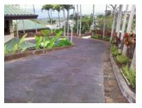
CONDITION: Good condition for age, Cracks noted are typical minor hairline type No lift or settlement
