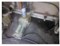
JET MOTOR/PUMP CONDITION: Newer, appears very good, replaced in 2011 as per disclosure. Motor runs smooth, no
