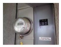
GROUND: Grounding system is present and appears O.K. UFER ground to slab.
