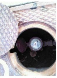
WATER METER FLOW DIAL: The Flow Dial at the water meter is dead still, indicating no leakage within the house
